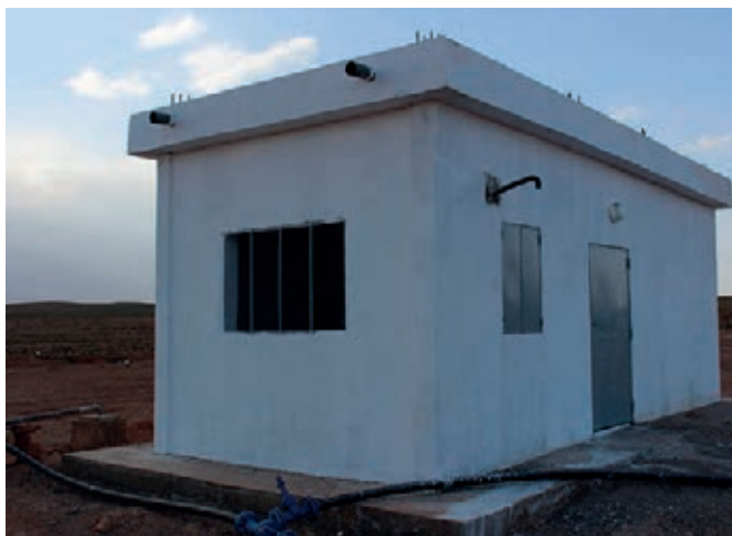
Pictured: The new water well
