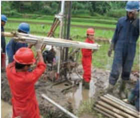
Figure 4: Preparing to set dynamite charge in the shot-hole.
